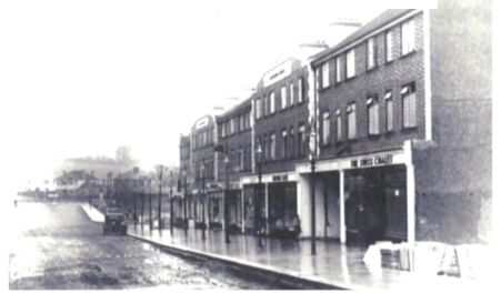
Very early, pavements being laid
